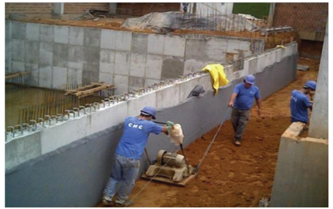
Fig 4.19: Installation of Geocomposite Drain
