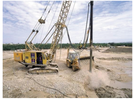
Fig- 2.4: Ground improvement using stone column
