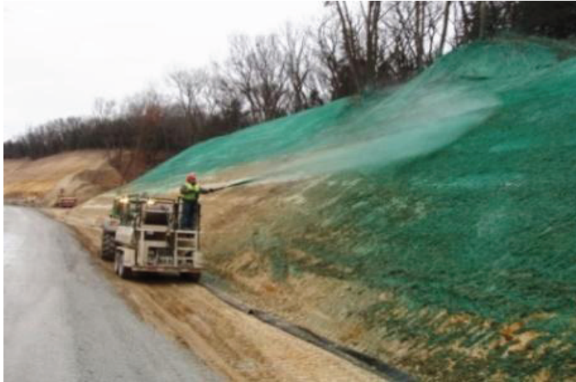
Fig-8.5 Figure showing Hydro-seeding/hydro-mulching on slope
