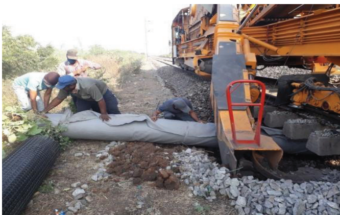
Fig-10.3(a): Insertion of Material under BCM
