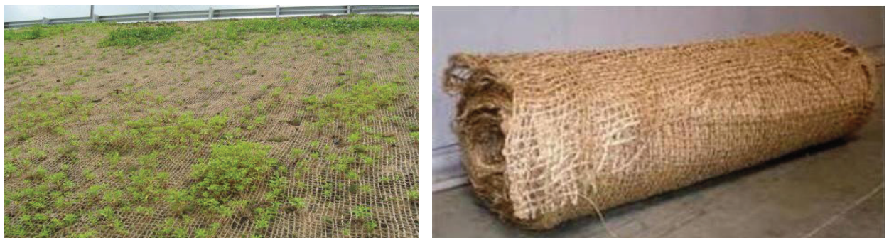
Fig-8.1 (a): Slope erosion control using Geo jute
