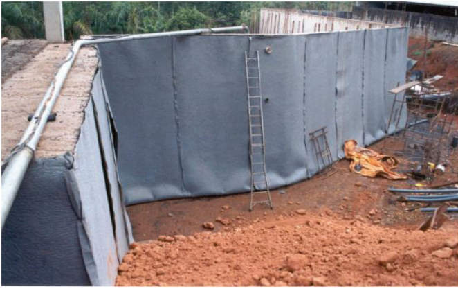
Fig 4.19: Installation of Geocomposite Drain
