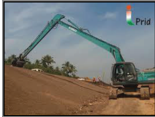
Fig-E3: Working of Slope Vibratory Roller
